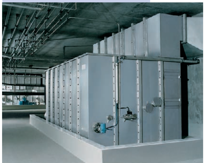
Jet scrubbers for the separation of colour mist from a paint shop for commercial airplanes. material: stainless steel 1.4571
